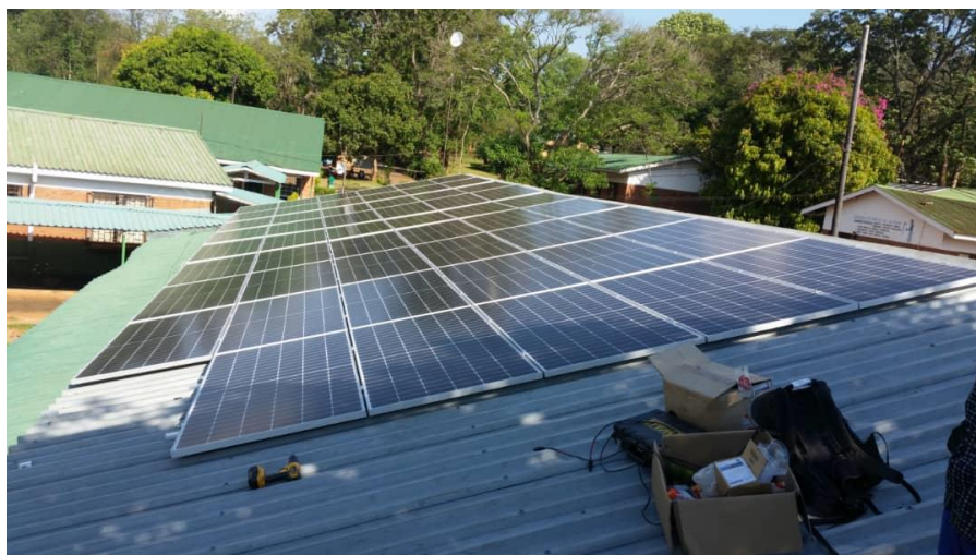
Installation of new solar panels on out-patient department
