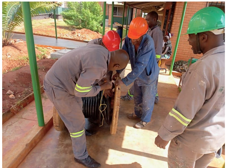
Laying underground cable to wards
