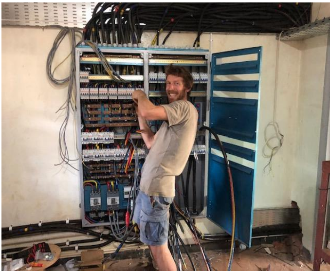
Michael Cocquyt working on new main board
