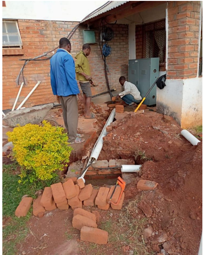
Maintenance team working on underground cable conduits
