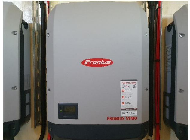
Fronius Symo solar inverter
