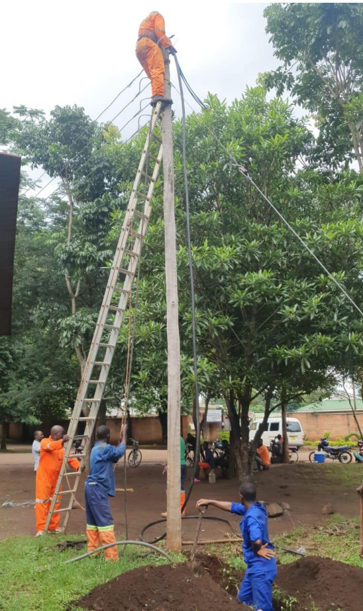
New, thick overhead line installation (over 200m)
