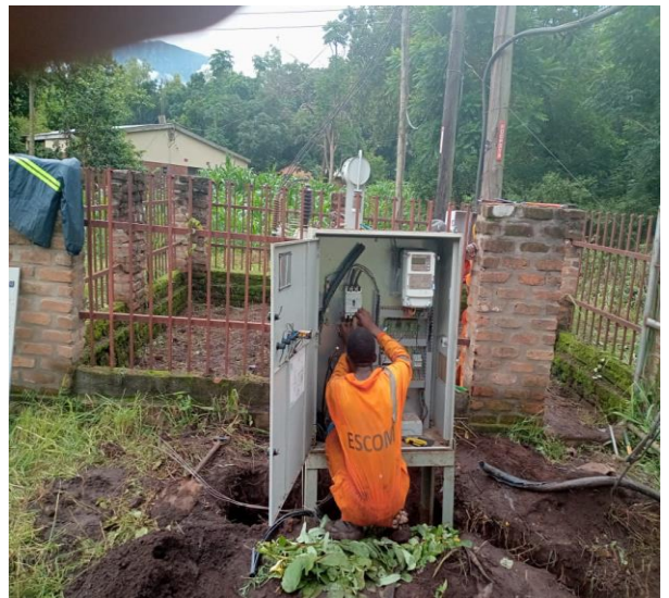
Transformer connection upgrade
