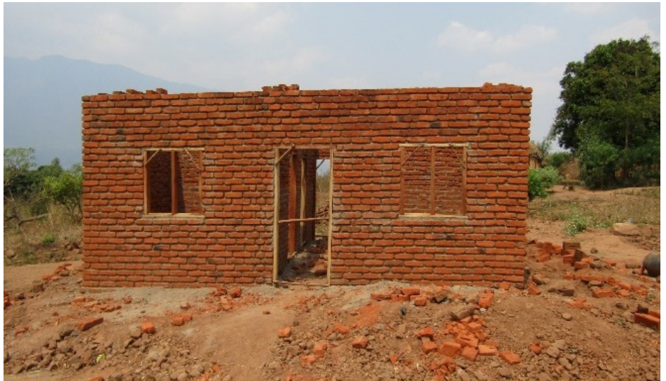
Construction of the new house at Khoviwa underway
