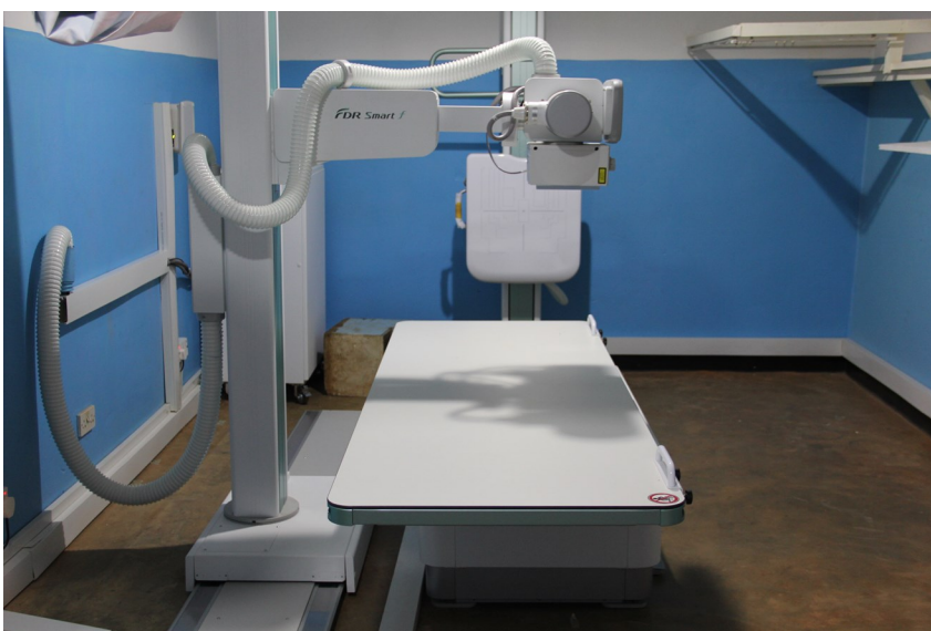
The refurbished X-ray room with new X-ray machine
